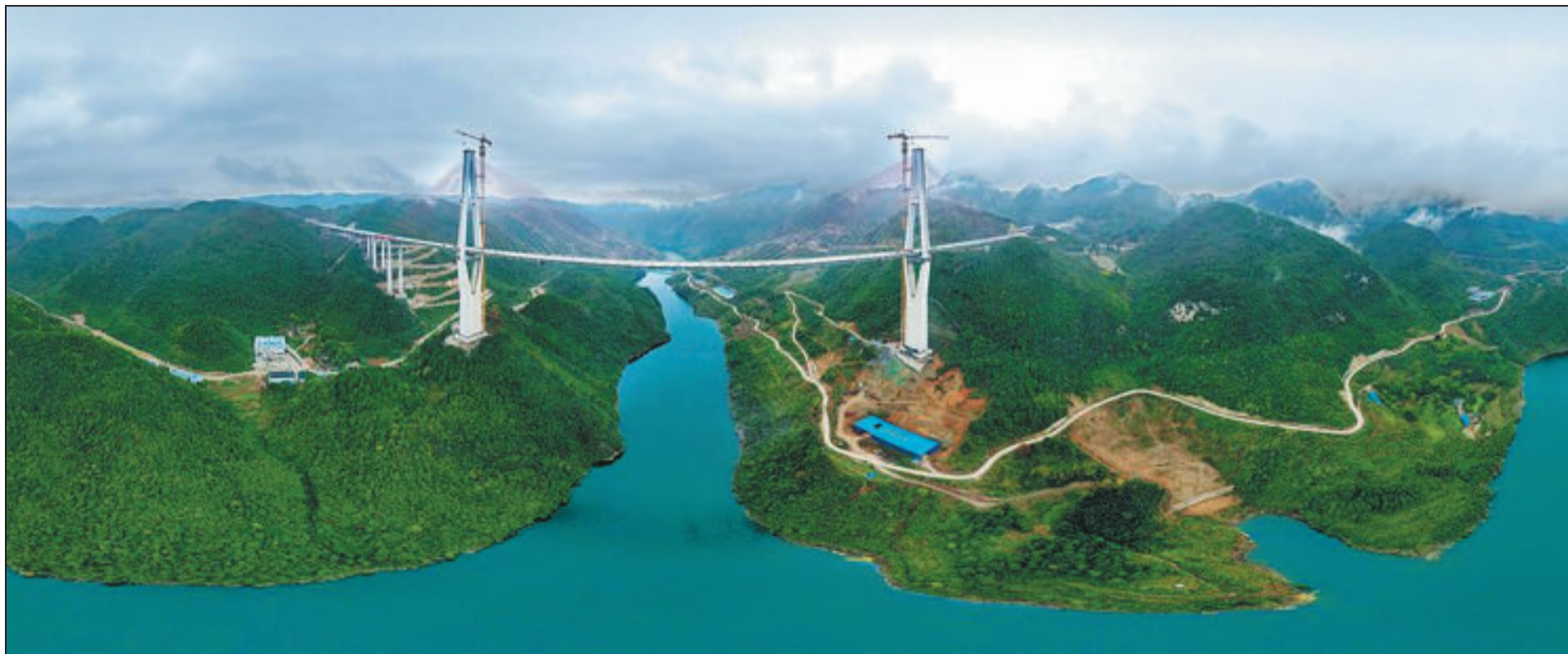
The Xiangjiang Bridge, in Guizhou province, stands one day short of completion in this aerial photo taken Wednesday. The bridge connects the city of Zunyi and Yuqing county and is more than 1.7 kilometers long with a main span of 560 meters. LIU XU / XINHUA
