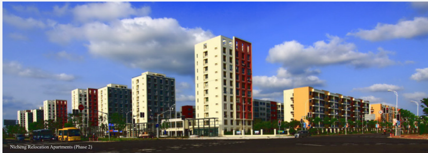
Nicheng Relocation Apartments (Phase 2)
