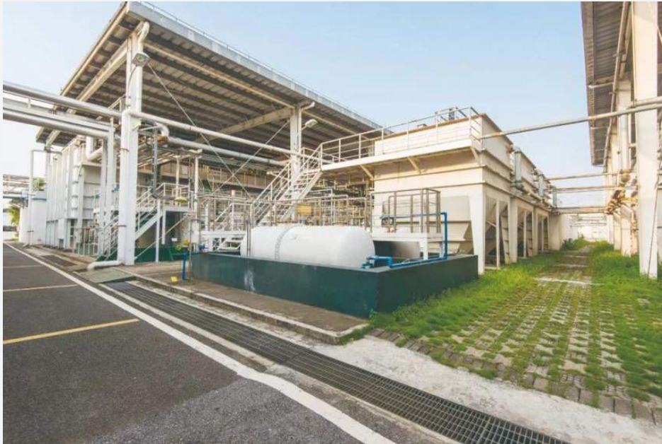
The GAC Honda wastewater treatment plant
