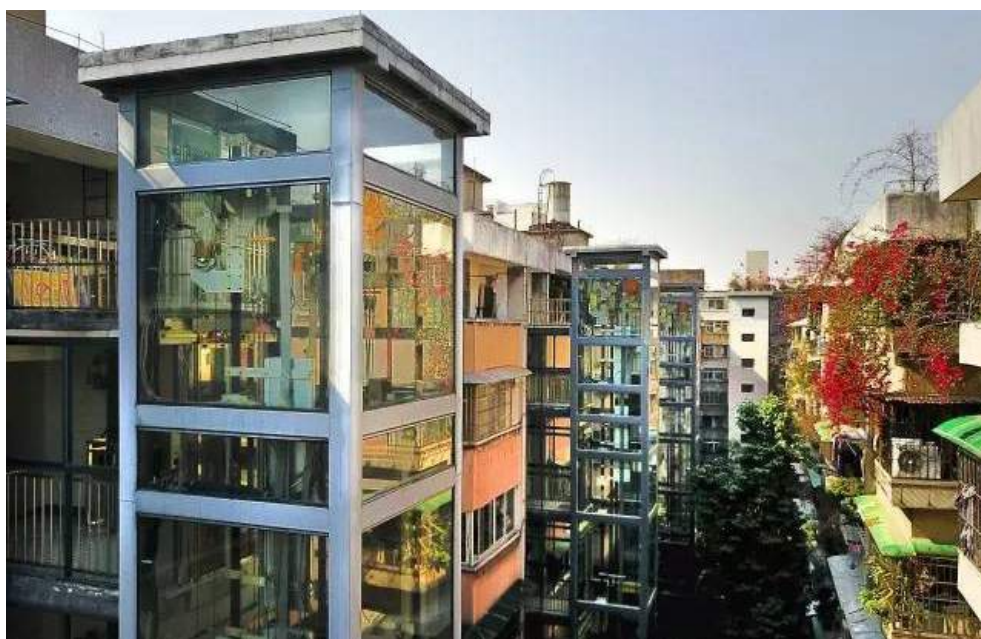
Installation of elevators in existing buildings
