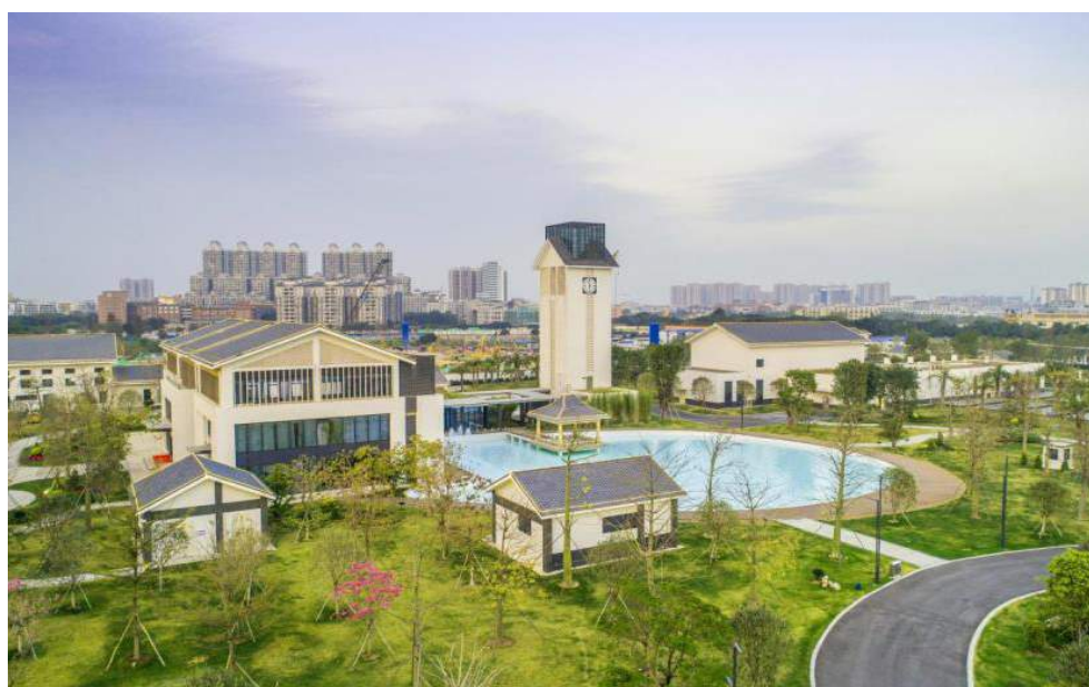
Wastewater purification facilities which have become part of the city landscape
