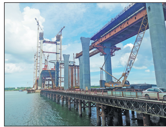
A cross-sea bridge is under construction in Zhanjiang.
