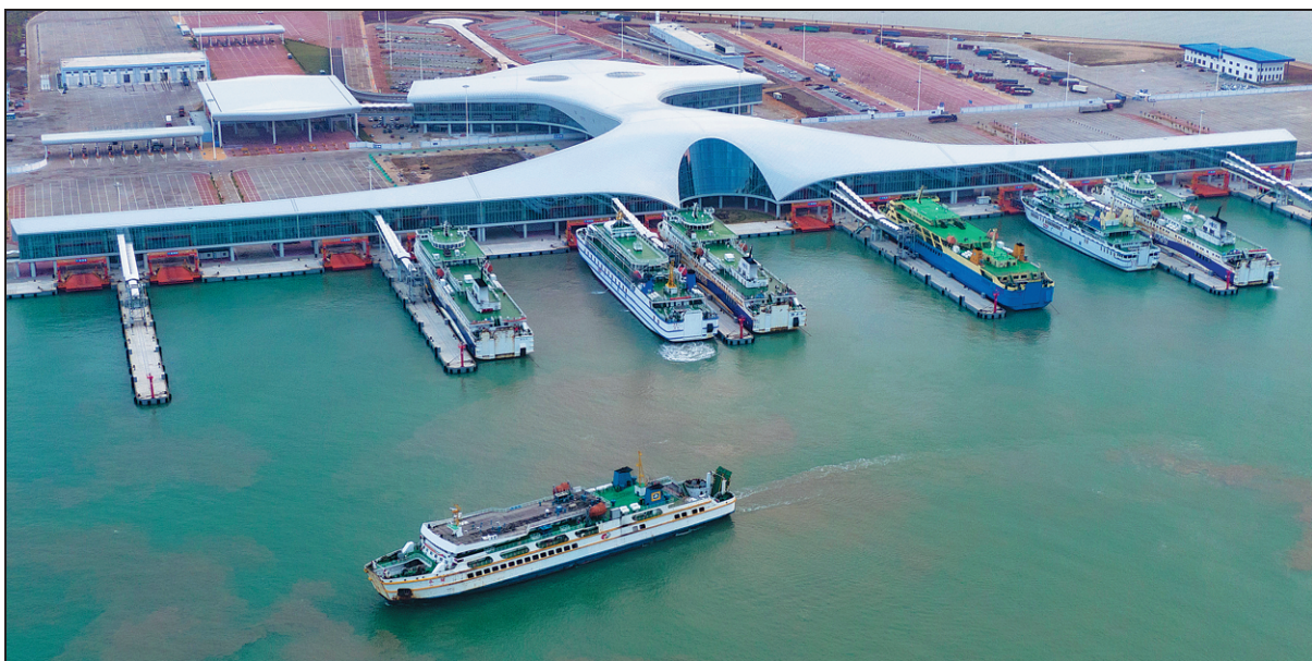
Ferries dock at Xuwen Port in Zhanjiang, Guangdong province. Xuwen Port has 16 ro-ro berths for 5,000-tonnage cargo and passenger vessels, and one 5,000-tonnage ro-ro berth specially designed for hazardous goods. PENG DECAI / FOR CHINA DAILY
