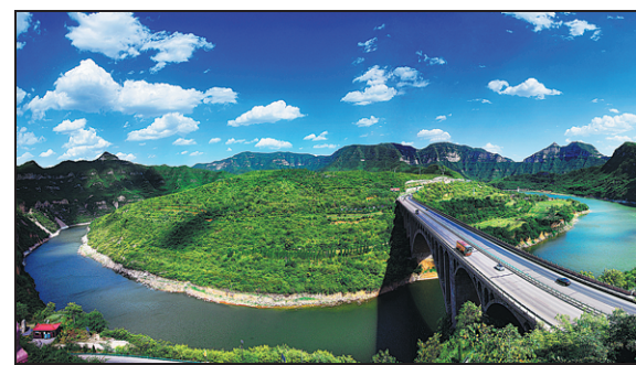
The Jincheng-Jiaozuo Expressway crosses the picturesque Danhe River valley in Jincheng city. WANG LIN / FOR CHINA DAILY
