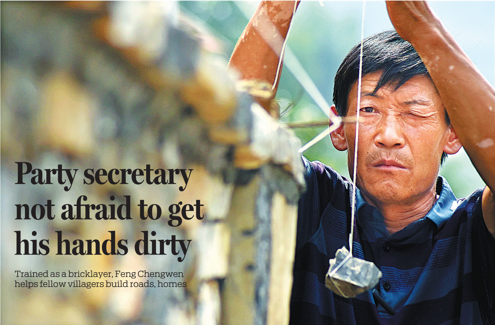
Feng Chengwen measures the verticality of a wall he built in Jibaoyu village in Yiyuan county, Shandong province, on Aug 10. PHOTOS BY ZHAO DONGSHAN AND FU YOUMIN / FOR CHINA DAILY
