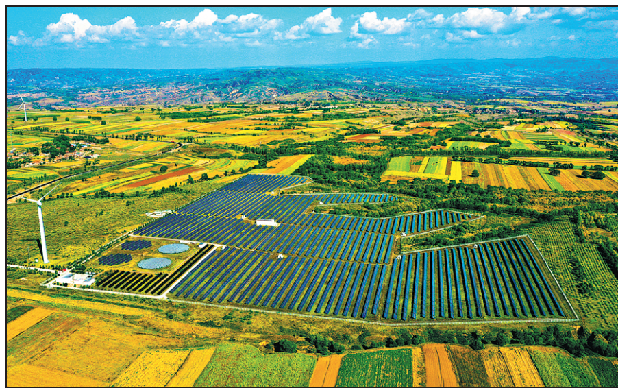
The 10-megawatt Youwei Solar Power Plant in Youyu county established by Jinneng Holding is the first solar power station in Shanxi province. TIAN ZHONG / FOR CHINA DAILY
