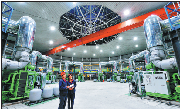
Technicians at Chengzhuang Thermal Power monitor the status of its coalbed methane-fired power generation equipment. QIU MEI / FOR CHINA DAILY
