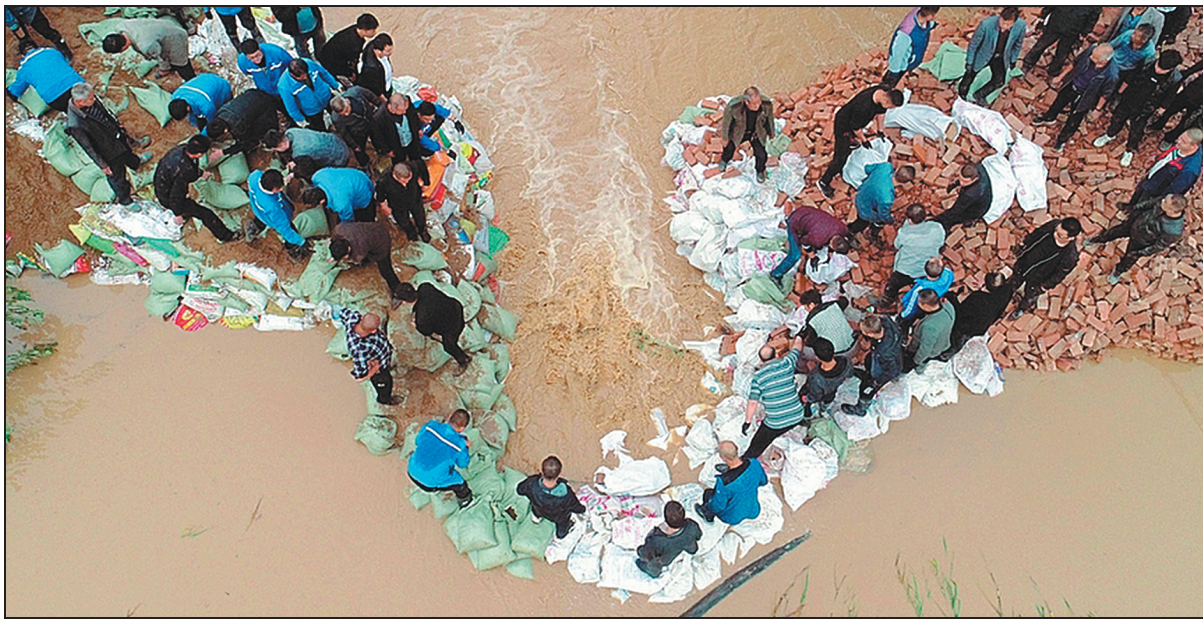
Rescuers in Jishan county repair a section of an embankment that was washed away by floodwaters of the Fenhe River. PROVIDED TO CHINA DAILY
