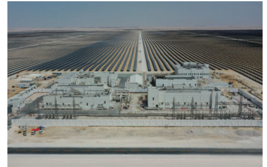
Alcazar PV Plant under Our General Contract
