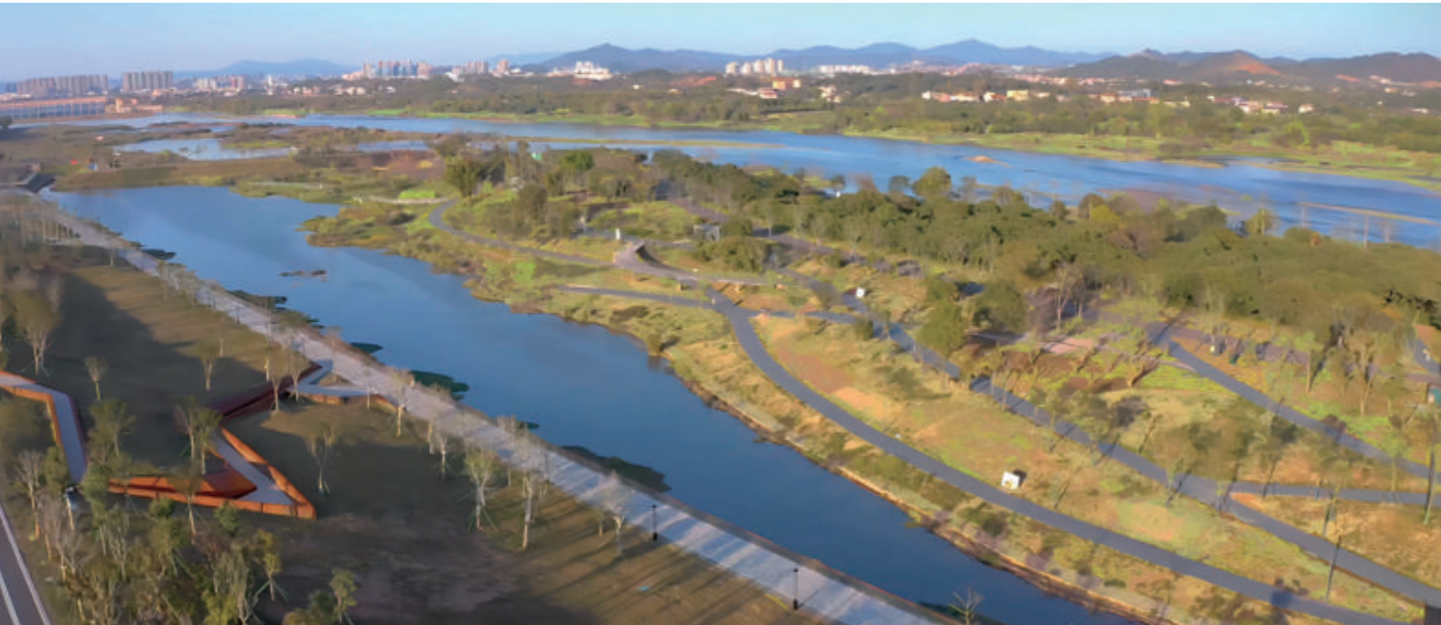
Aerial Photo of Heyuan Egret Island Eco-Park in Guangdong
