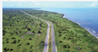
Nzeto-Soyo Highway Construction Project in Angola
