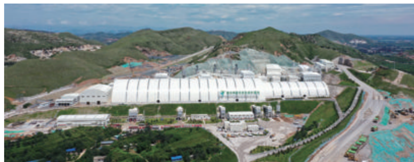
Extra-large green sand and gravel base in Xiong'an New Area
