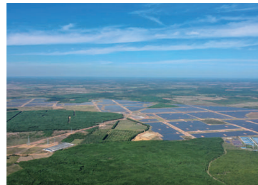
Loc Ninh 550 MW PV EPC Project in Vietnam
