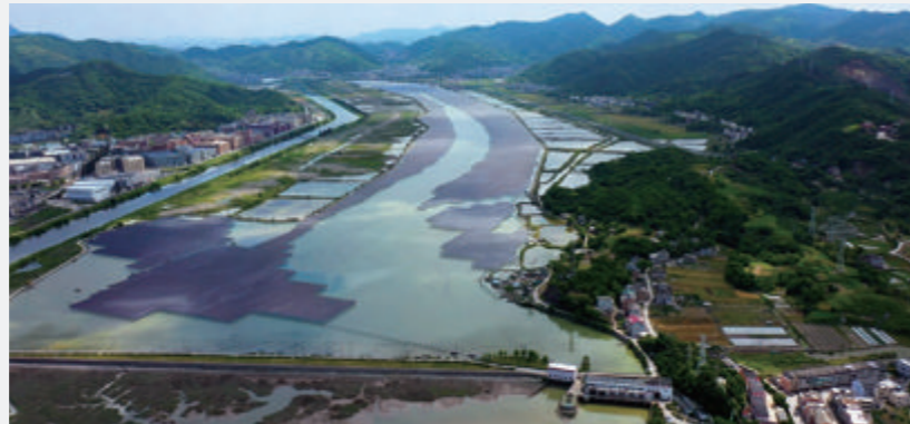
Wenling 100 MW Tidal-Photovoltaic Hybrid Power Station in Zhejiang, the first tidal-photovoltaic hybrid power station in China
