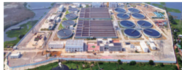
Sewage Treatment Plant in Dasherikandi, Bangladesh
