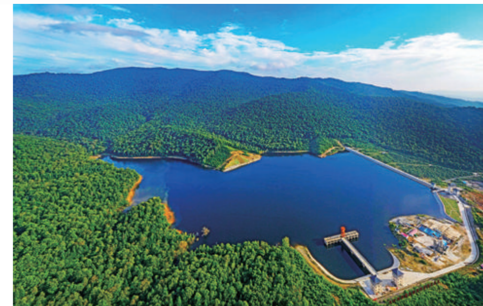
Dunhua Pumped Storage Power Station in Jilin - the first 700-meter-head pumped storage power station designed, manufactured, installed, commissioned, operated and managed completely independently in China
