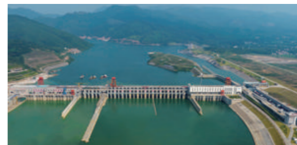
In November 2022, the first unit on the right bank of Dateng Gorge was put into operation
