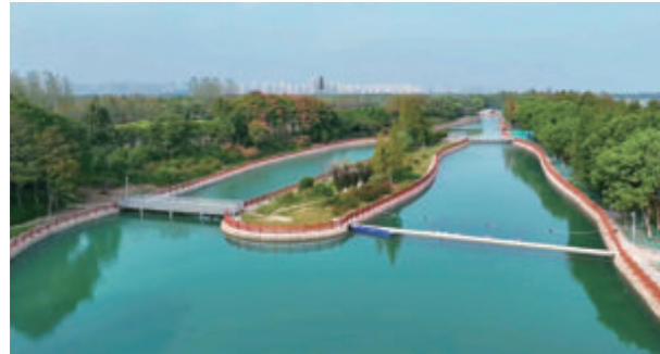
POWERCHINA's first cyanobacteria treatment project - Zhangqiao Port In-situ Algae Control Pilot Project
