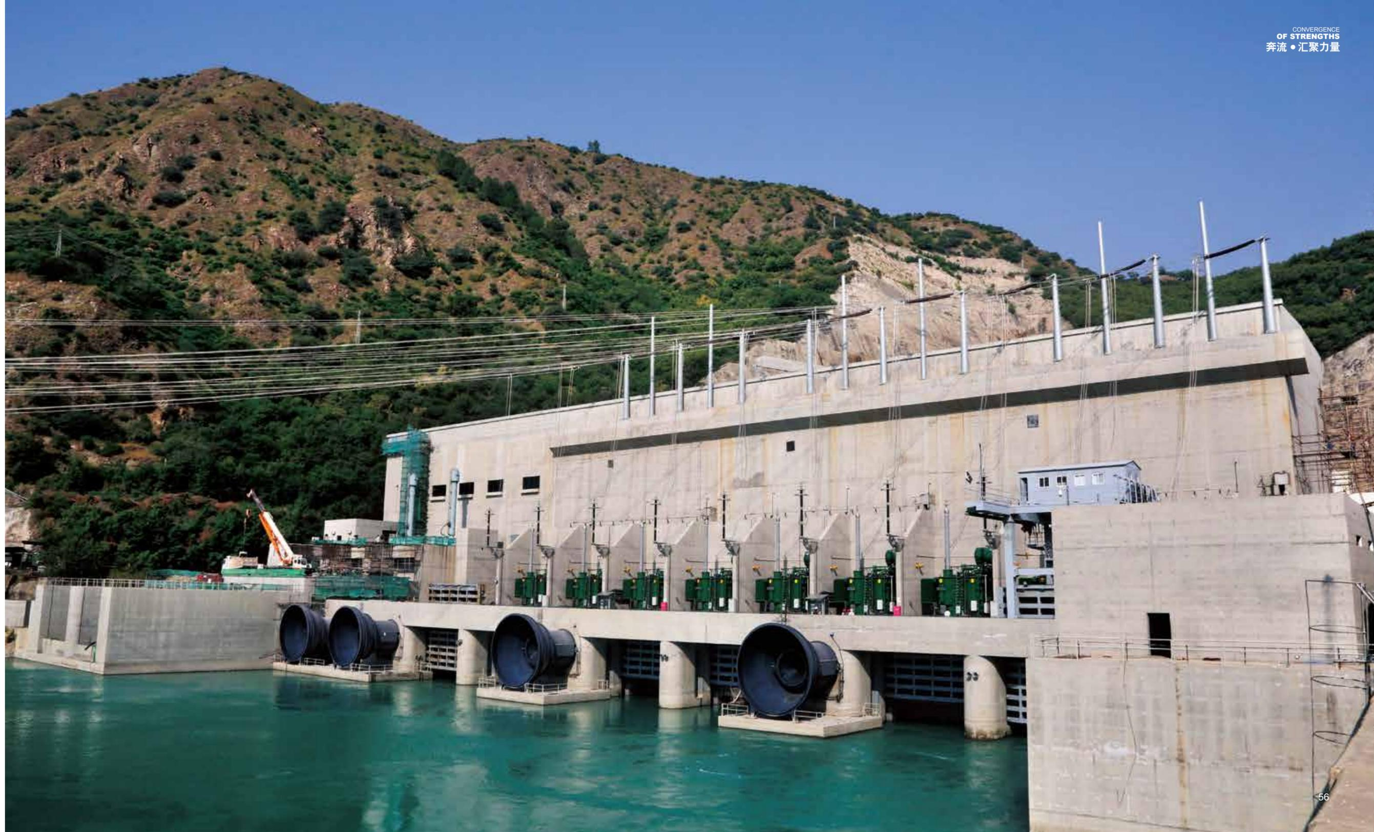
The Tarbela dam is a comprehensive water conservancy project on the Indus River, 120km from the capital Islamabad. Tarbela 4th Extension Hydropower Project upgraded the existing power station by adding three German 470MW Francis turbines to increase the installed capacity from 3478MW to 4888MW. The project employer is Pakistan Water and Power Development Authority (WAPDA).
